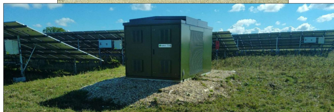
Figure 26 : Illustrations photographiques des structures (source : COMIREM SCOP)
